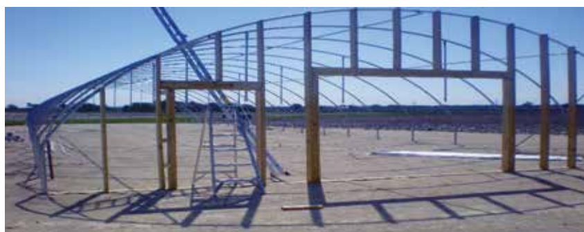
Construction of the Walnut Grove Farm Greenhouse
